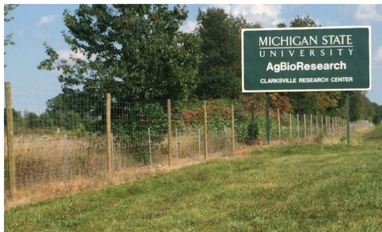
Deer fence installation completion.
